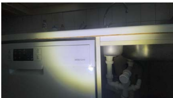
Svelling underkant benkeplate
