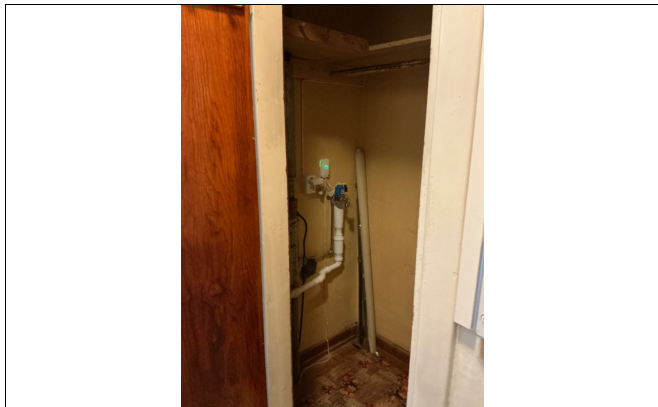
Opplegg for vaskemaskin i kott
