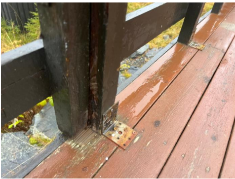
Begrenset innfesting utsatt for sideforskyving
