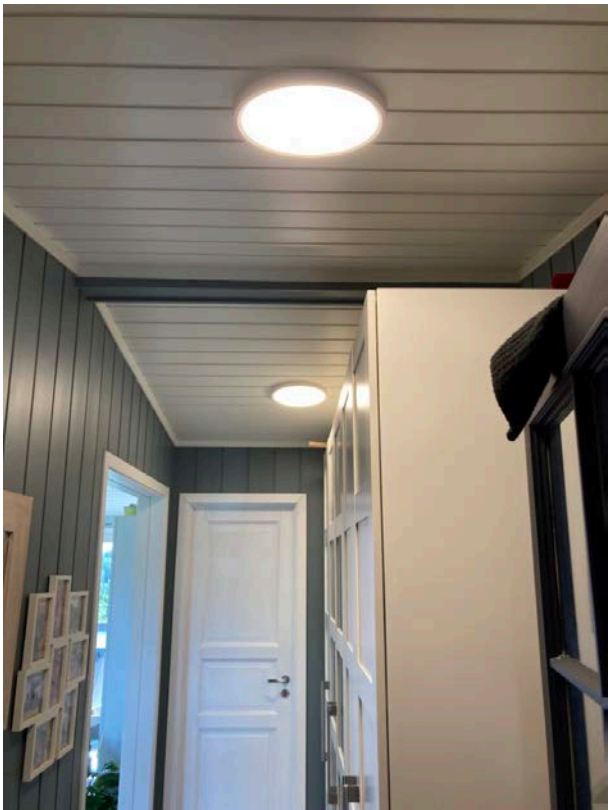
Nye lamper montert. Ok
