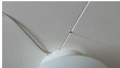
Synlig innfesting i himling.
