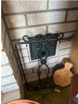
Mangler ildfast plate under sotluke.
