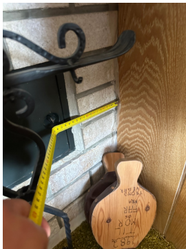
Mangler ildfast plate under sotluke.
