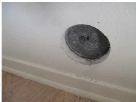
Hulltaking i utfored vegg
