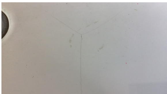
Riss i servant.
