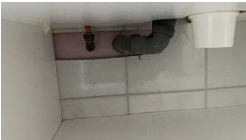
Hull i baderomsplate under vask
