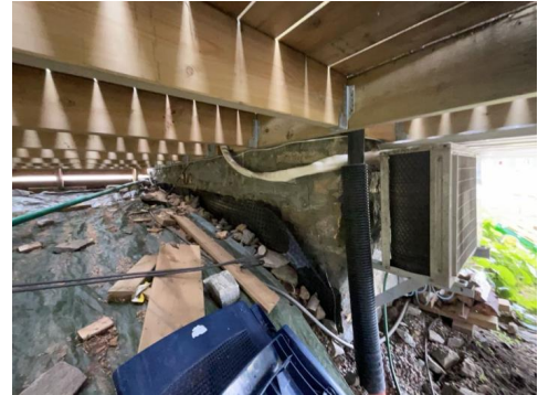
Mur sett under veranda
