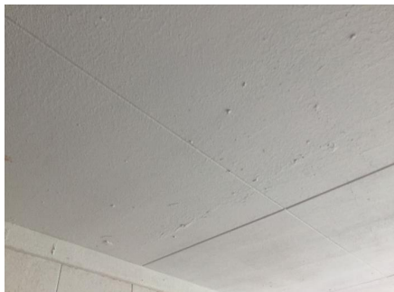
Grov overflate i himling.
