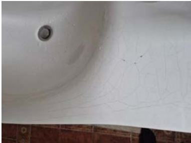
Krakelering i servant.
