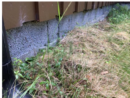
Mangler puss/slamming.
