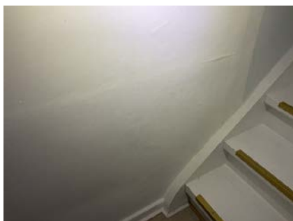
Overflate i trapperom.
