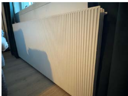
Eldre radiatorovn i stue.
