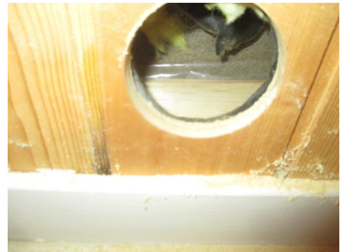
Hulltaking i utfored vegg.
