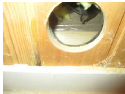
Hulltaking i utfored vegg.
