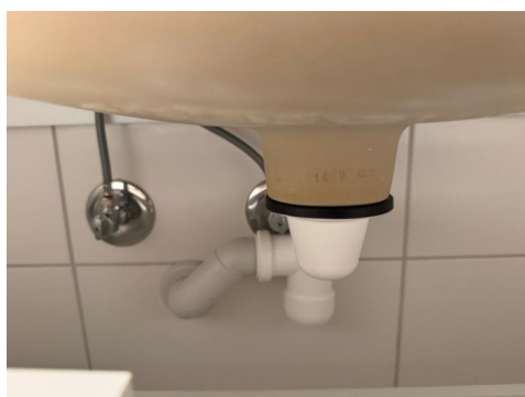
Røropplegg under servant.
