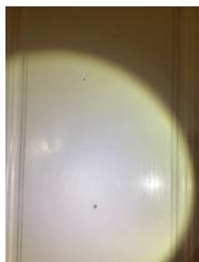
Noen små skruer hull i to fronter.
